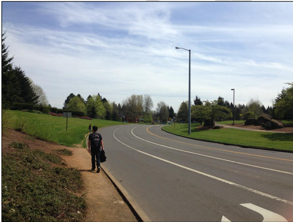
Figure 21 An incomplete sidewalk network on CCC Oregon City at the OR-213 entrance
